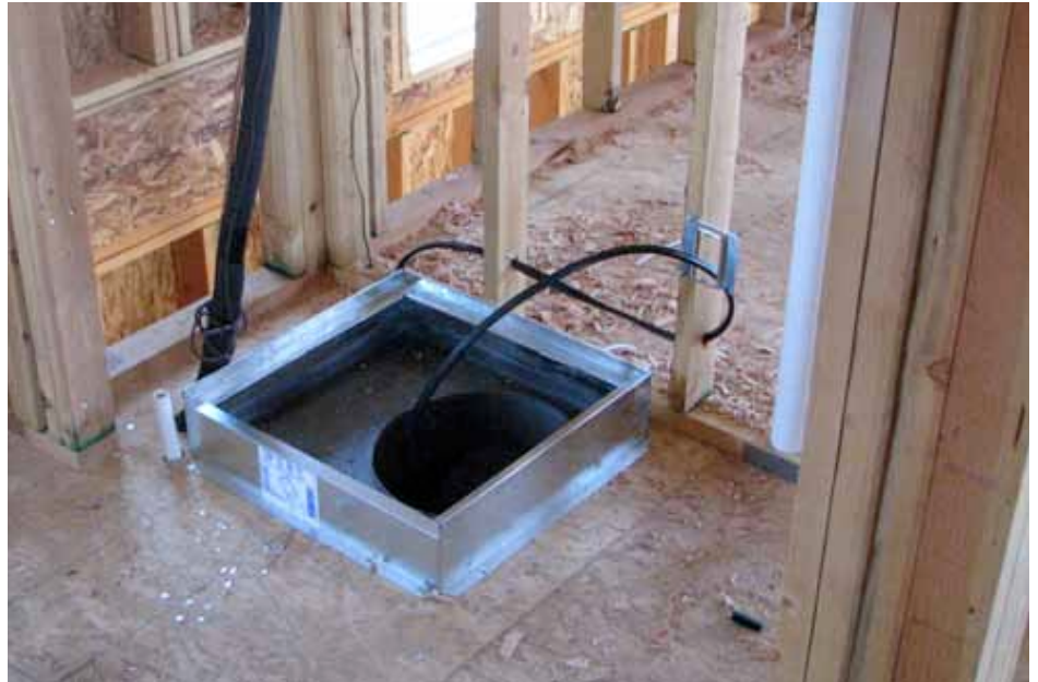
2nd floor closet plumbed to receive air handler.
