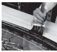
10. Wipe off excess stain. Use the 3" brush as a scoop at a sharp angle. Make sure to get inside the grooves as well as flat surfaces. After each pass, wipe the brush on a rag to keep clean.
