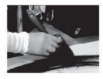
12. Use the 3" brush to smooth out the stain. Using a back and forth motion will help get stain into all of the grain. Pay special attention to the corners and the small, detailed parts of the embossment.
