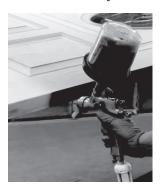
5. Tilt the door at a 45° angle, then continue spraying using a continuous left-to-right, right-to-left motion.
