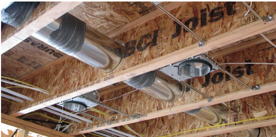
Boise Cascade Conditioned Air HVAC framing system installation summer 2010 in Central Point, Oregon by Vision Homes of Medford, Oregon. HVAC work by Spring Air Heating & Cooling, Inc. of Jacksonville, Oregon
