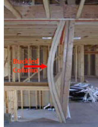
Figure 1: Column Buckling
